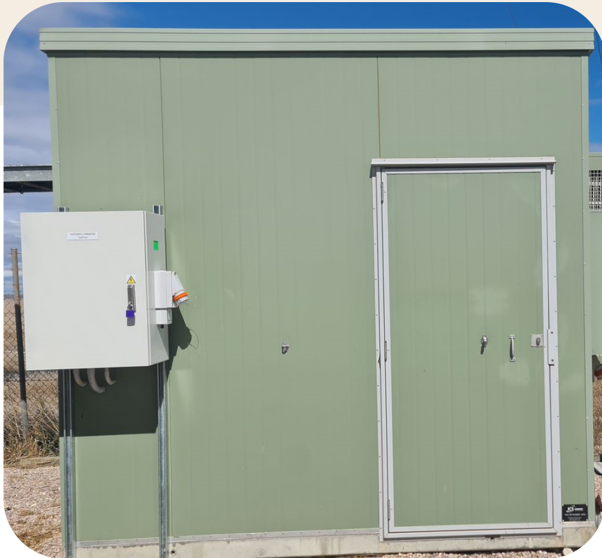
Automatic Transfer Unit (ATU)
